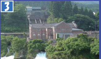
▲Fukuoka Dai-ichi Power Plant The first power plant that utilized the Tedori River, built in 1911.
